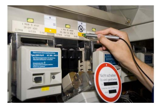
V-RFID chips of Evonik to indicate equipment deactivation due to ongoing work
