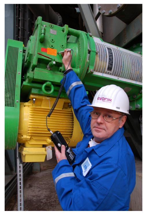
Usage of RFID-chips for maintenance
